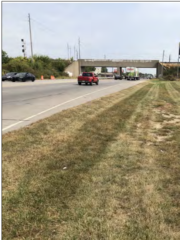
Picture 5—Project interior and railway crossing east view; 17 SEP 2020.
