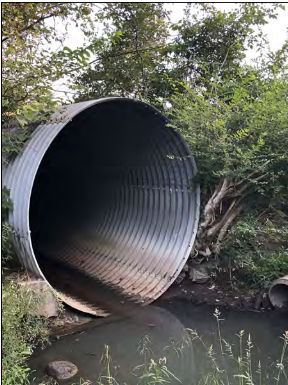
Picture 3—Shiloh Creek; northeast view; 17 SEP 2020.
