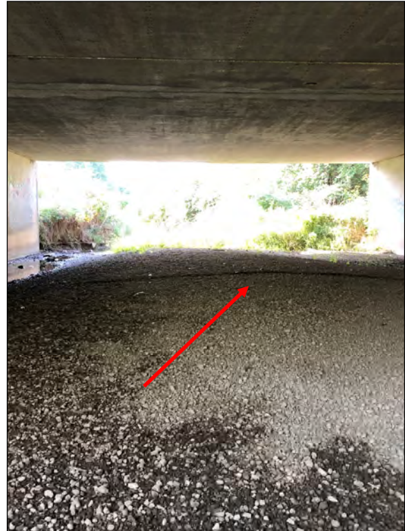
Picture 2— Center span—note line of guano at bridge center; 17 SEP 2020.
