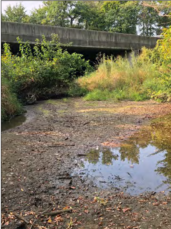
Picture 1—Southwest view of bridge; 17 SEP 2020.
