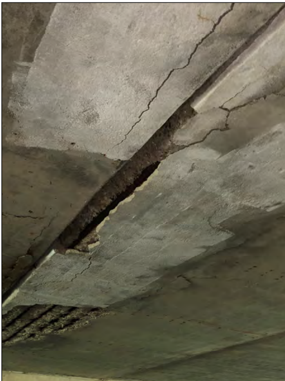
Picture 11—East span ceiling; 17 Sep 2020.
