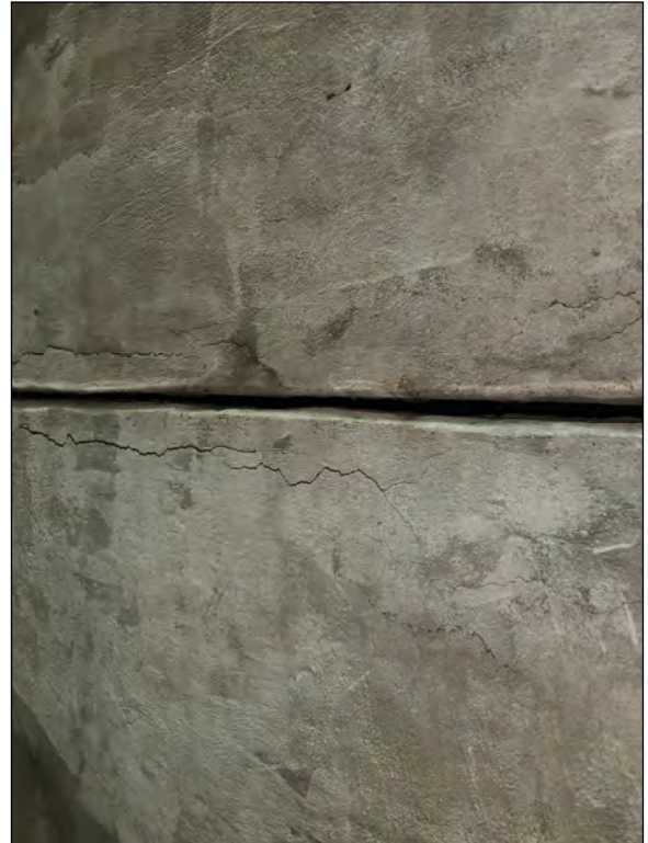
Picture 10—West span ceiling; 17 SEP 2020.
