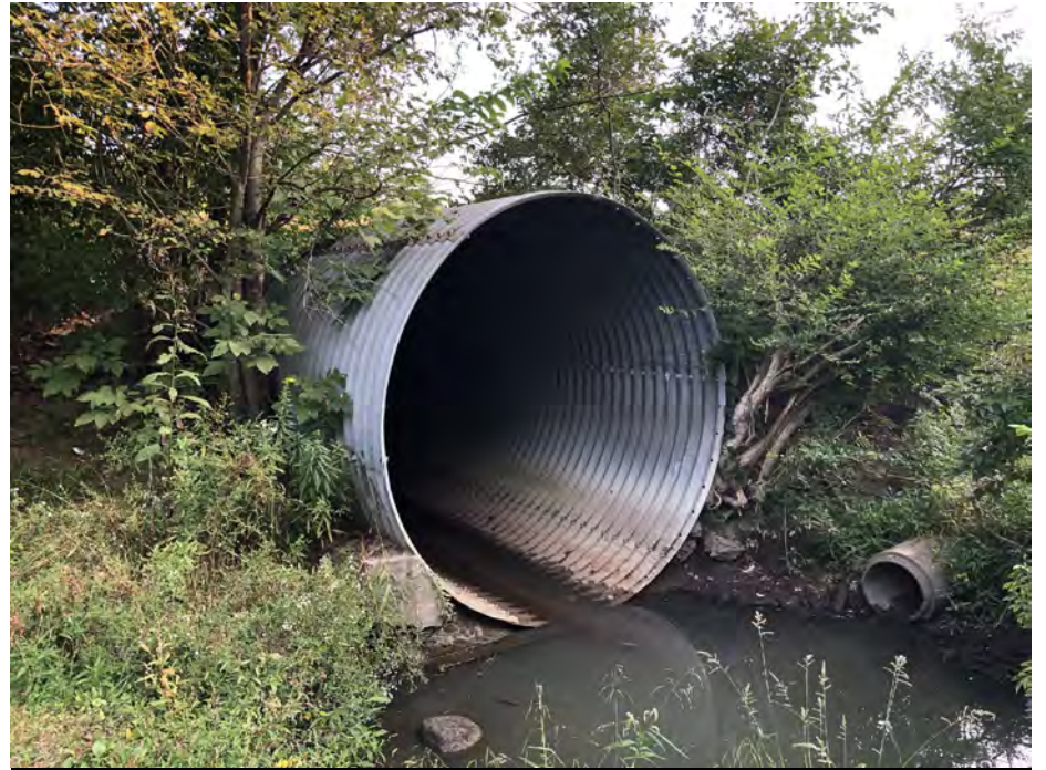
Photo 38- Shiloh Creek Culvert Northeast View, (Map 2) - 17 SEP 2020
