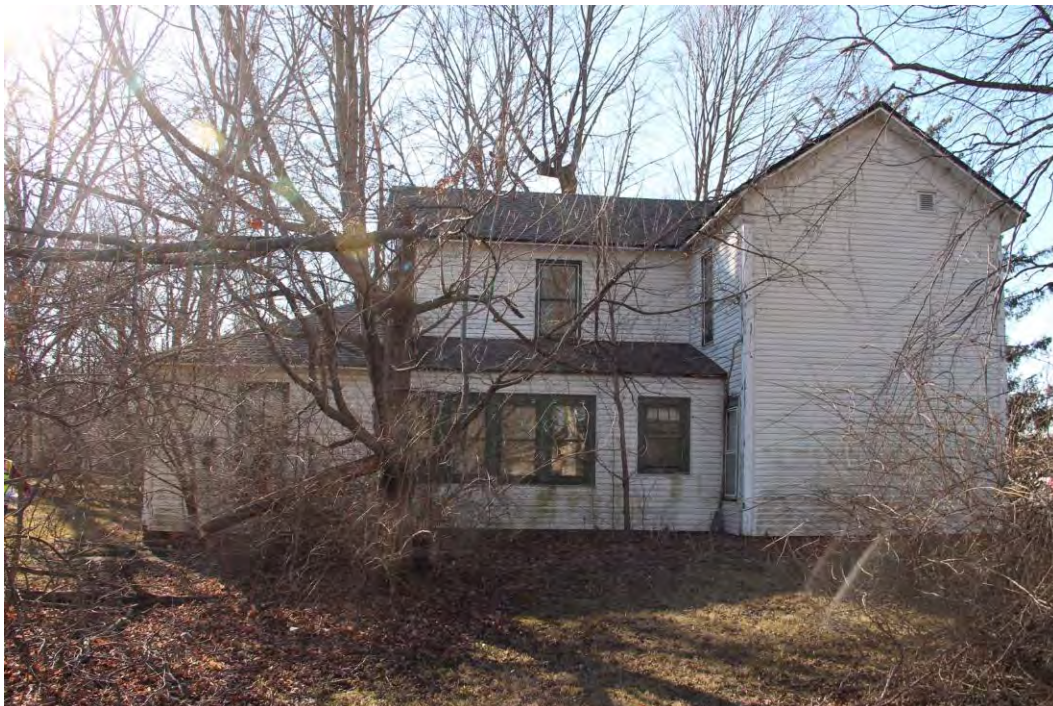
Photo D-6. IHSSI # 097-117-56005, 9055 Rockville Road, east (side) façade, facing west.
