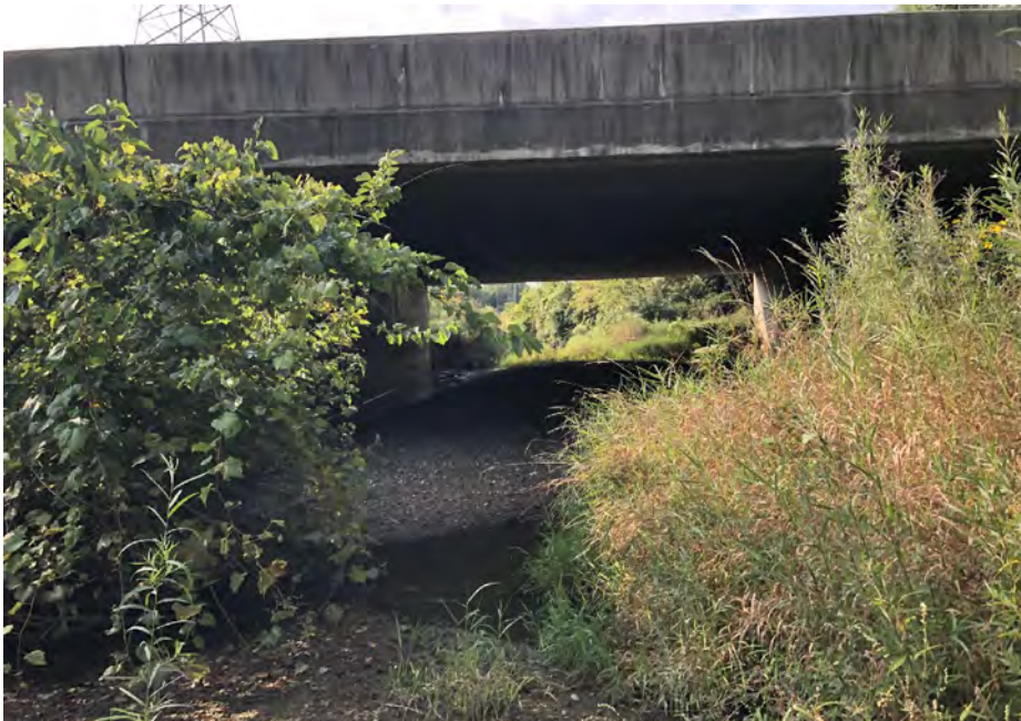
Photo 131- East Fork White Lick Creek Structure South View, (Map 5) - 17 SEP 2020
