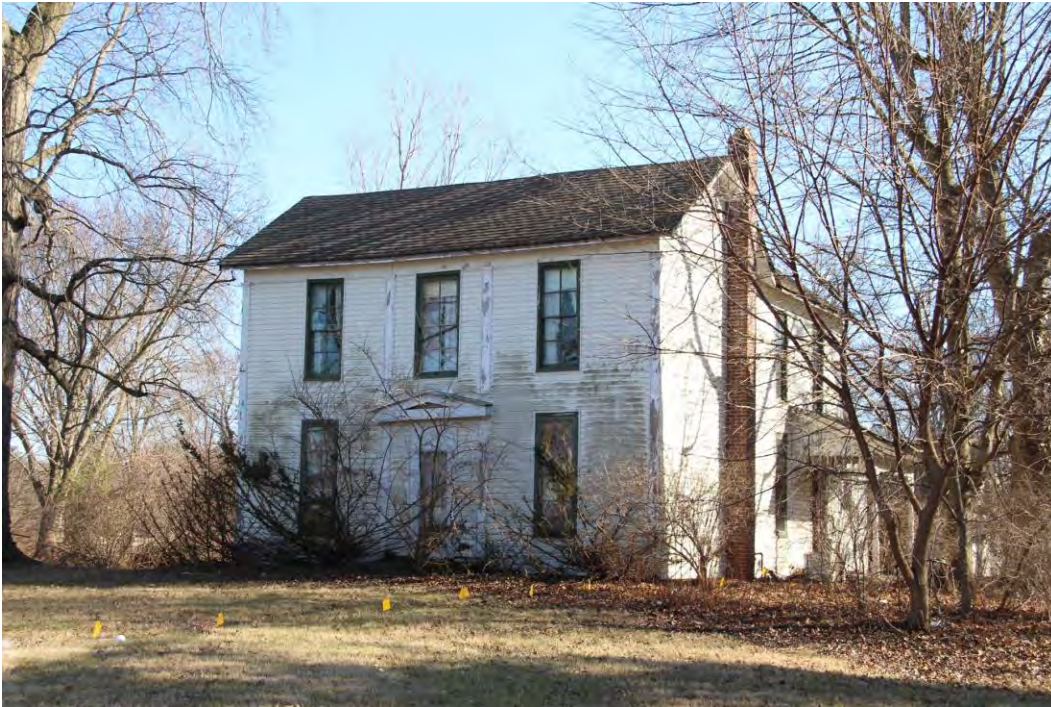
Photo D-3. IHSSI # 097-117-56005, 9055 Rockville Road, north (front) and west (side) façades, facing southeast.
