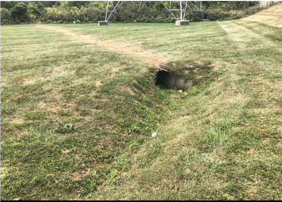
Photo 127- RSD4 Culvert, Southwest View, (Map 5) - 17 SEP 2020
