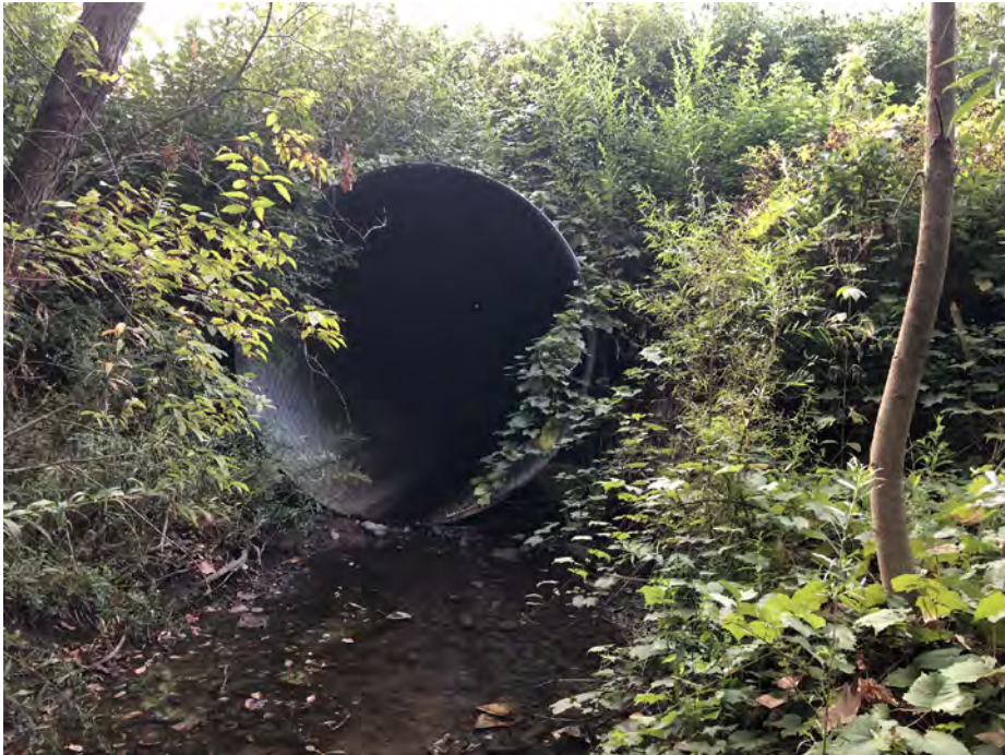
Photo 29- Shiloh Creek Culvert Southeast View, (Map 2) - 17 SEP 2020
