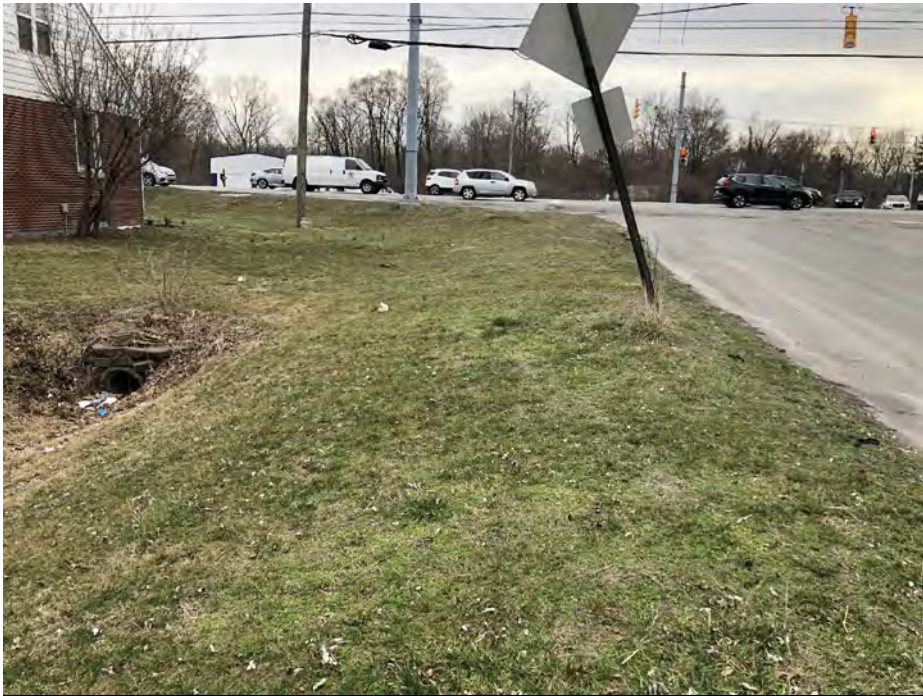
Photo 71- RSD10 South View- 12 MAR 2021
