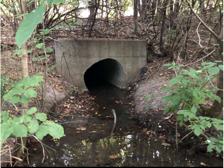
Photo 26- Shiloh Creek Pipe Northeast View, (Map 2) - 17 SEP 2020
