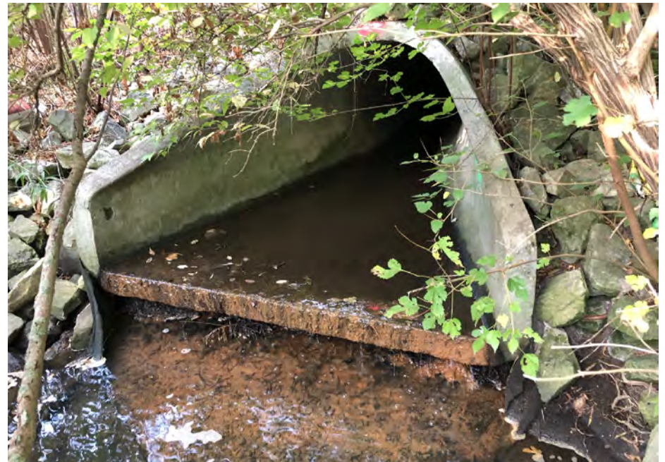
Photo 36- UNT1 to Shiloh Creek Culvert Southwest View, (Map 2) - 17 SEP 2020
