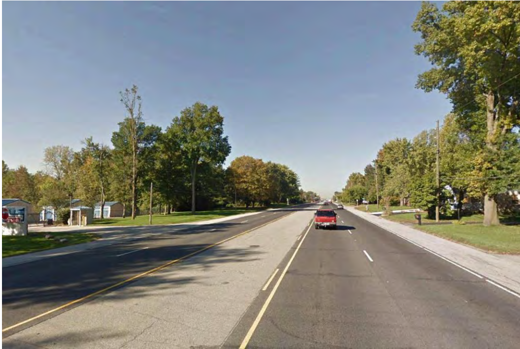
Photo D-17. Streetscape from a location near 8530 Rockville Road, facing west.
