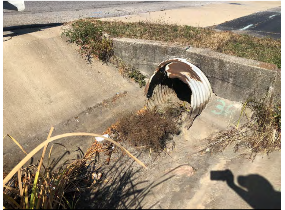
Photo 238- JAR1 Culvert, (Map 10) - 7 OCT 2020
