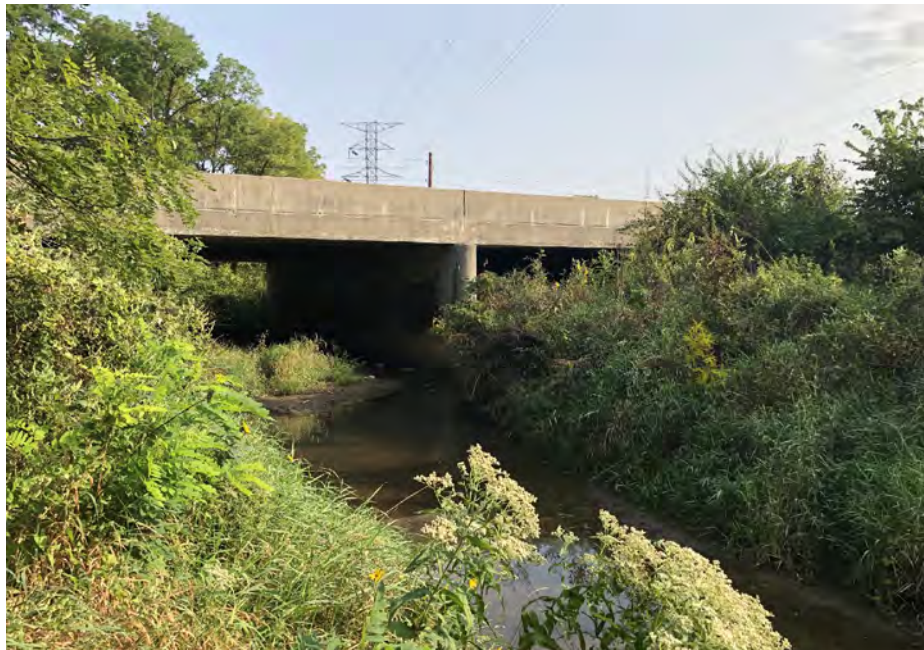
Photo 135- East Fork White Lick Creek Structure Northeast View, (Map 5) -17 SEP 2020
