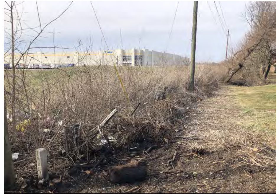
Photo 210- US 36 North Side Utility Easement, Northwest View- (Map 9) 12 MAR 2021
