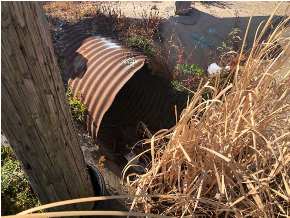
Photo 239- JAR1 Culvert, (Map 10) - 7 OCT 2020
