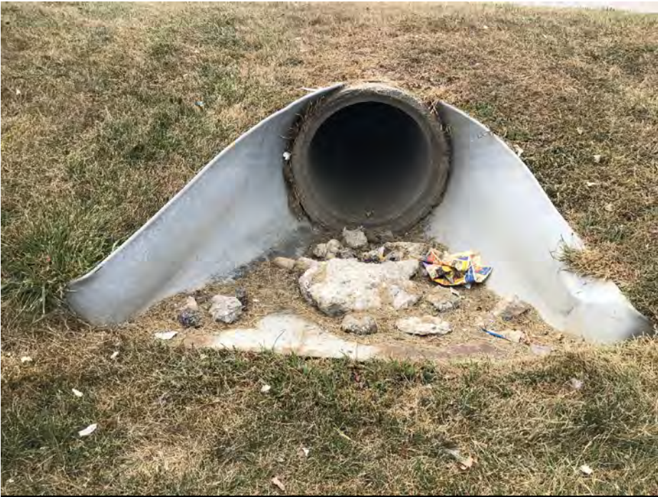
Photo 153- RSD4 Culvert, West View, (Map 6)- 17 SEP 2020
