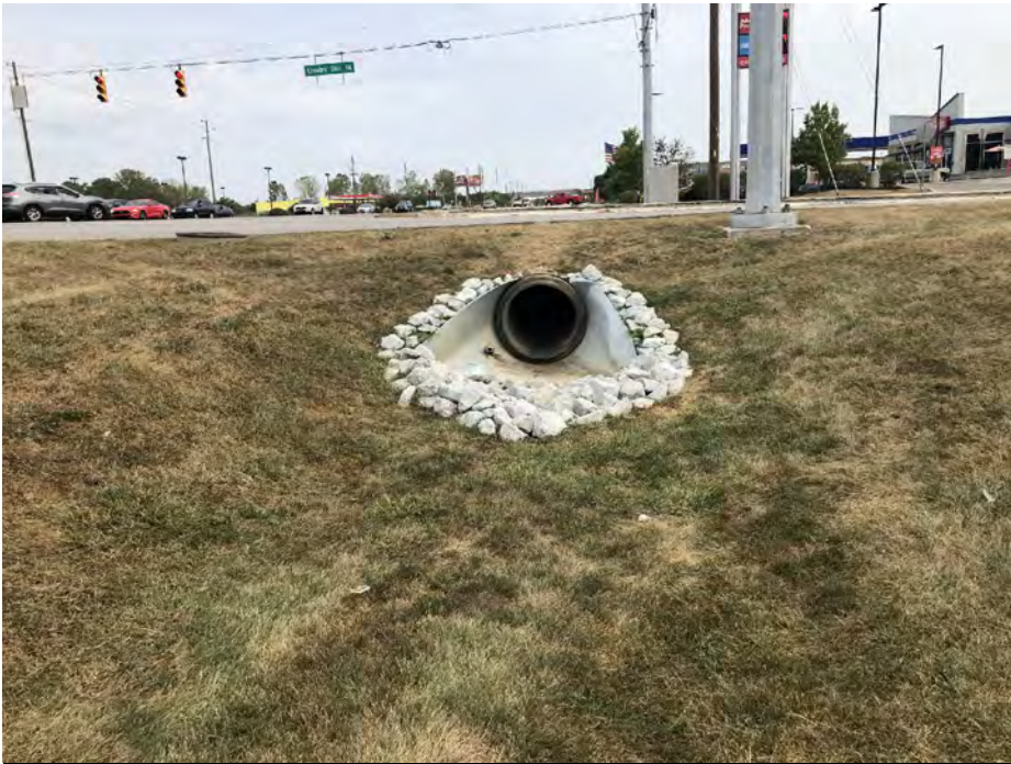
Photo 156- RSD4 Culvert, East View (Map 6)-- 17 SEP 2020
